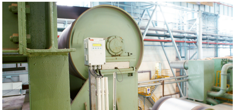
Large PillowBlock Tensiometers in a steel processing line.
