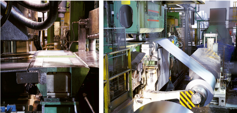
Millmate Strip Scanner and Stressometer Flatness Control System in a temper mill.
