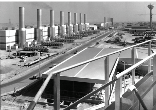
Gas fired turbine power plant
