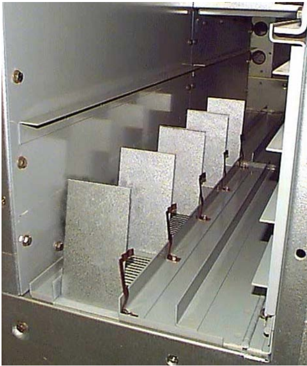
Breaker module ventilation vanes for Type 2BC
