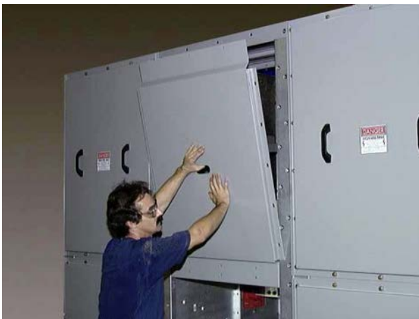
Installation of upper inner rear panel
