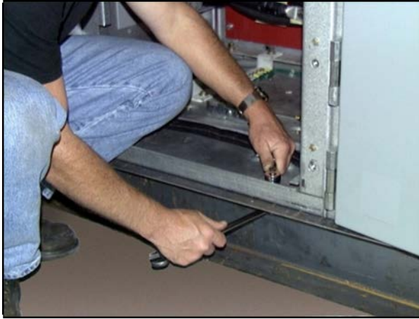
Unbolting the shipping bases
