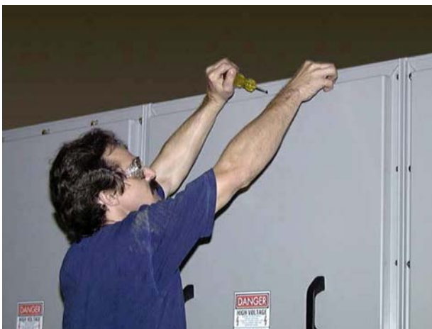
Installation of upper exterior rear panel
