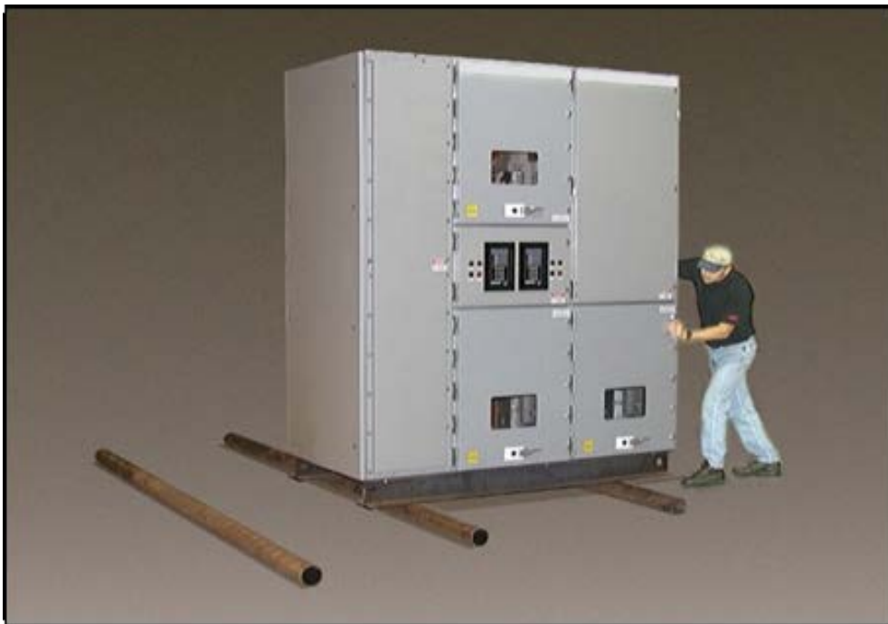
Movement of the frames with rollers
