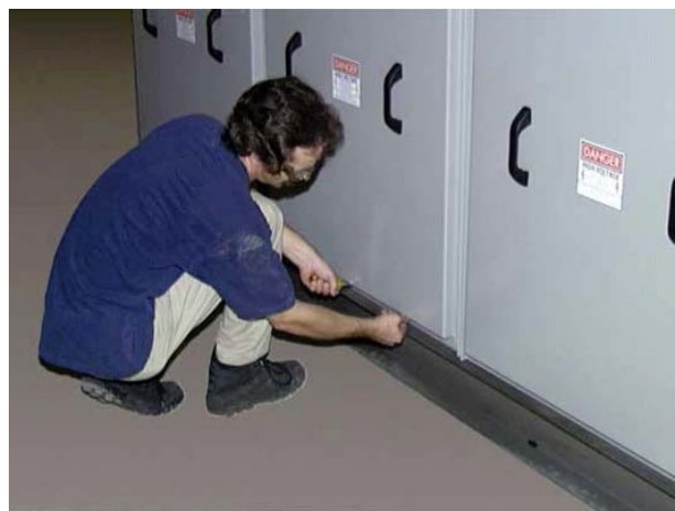
Installation of lower exterior rear panel
