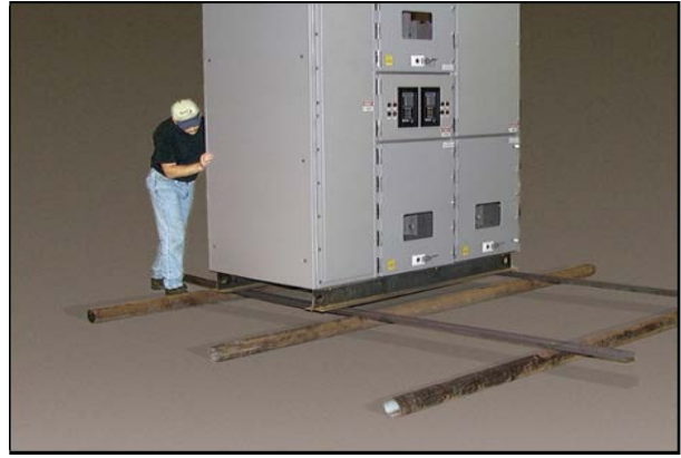
Lateral movement of the frames with rollers
