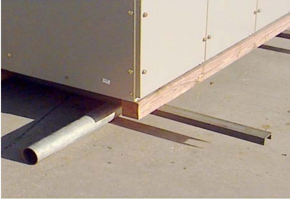
Position rails as shown for lateral movement
