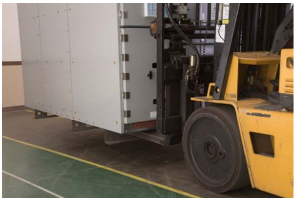
Lifting of switchgear frames with forklift
