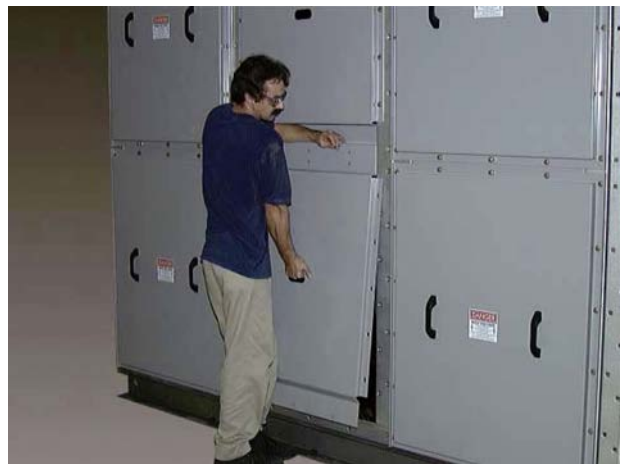
Installation of lower inner rear panel
