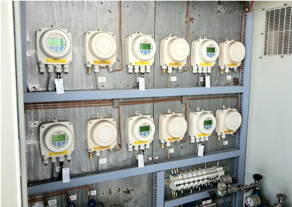
Endura AZ20 combustion gas analyzers in situ
